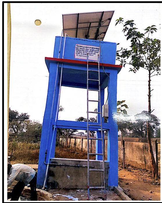
Solar Water Project in Tola
